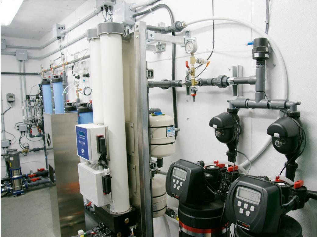
*The main treatment plant with GreensandPlus filter vessels on the right. The older Seccua UF system has been replaced by the new UF building*
