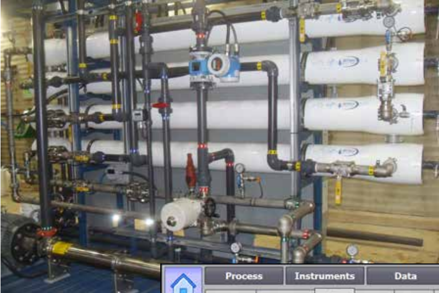
Above: The RO system uses energy recovery to save significant power costs.
