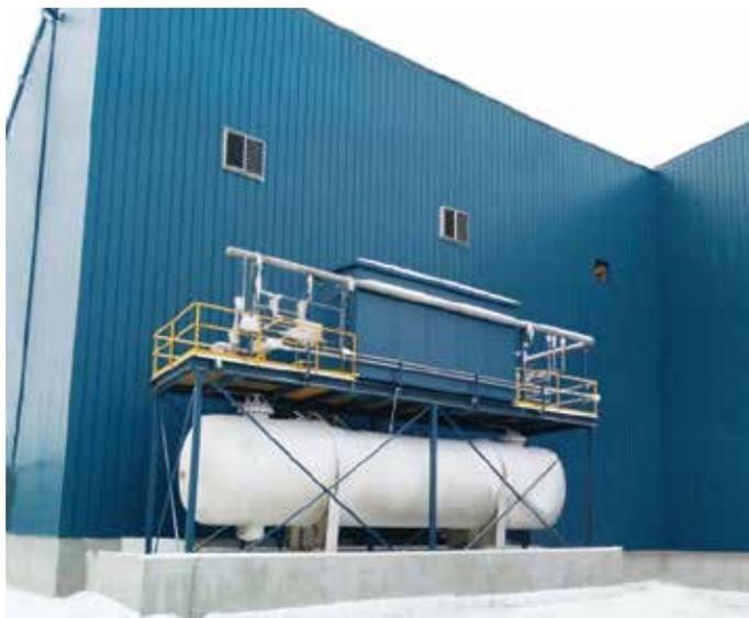
*The liquid SO<sub>2</sub> control building with storage tank located at Phoenix Gold mine (above), and the portable insulated gas handling building built at the Process Manufacturing factory*
