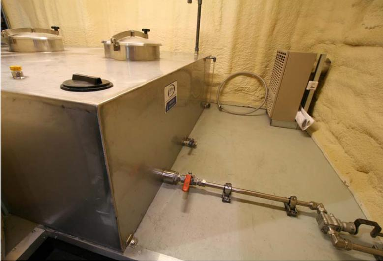
*Stainless steel water tank and propane heater inside the insulated container*
