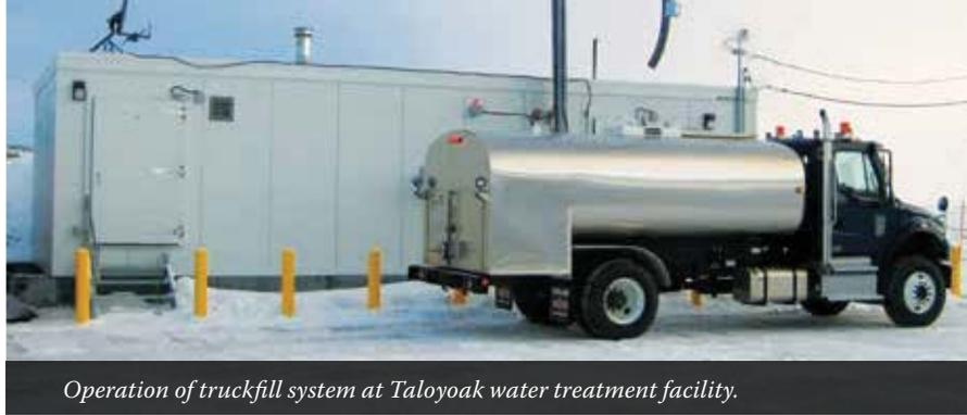
Operation of truckfill system at Taloyoak water treatment facility.
