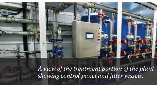
A view of the treatment portion of the plant showing control panel and filter vessels.
