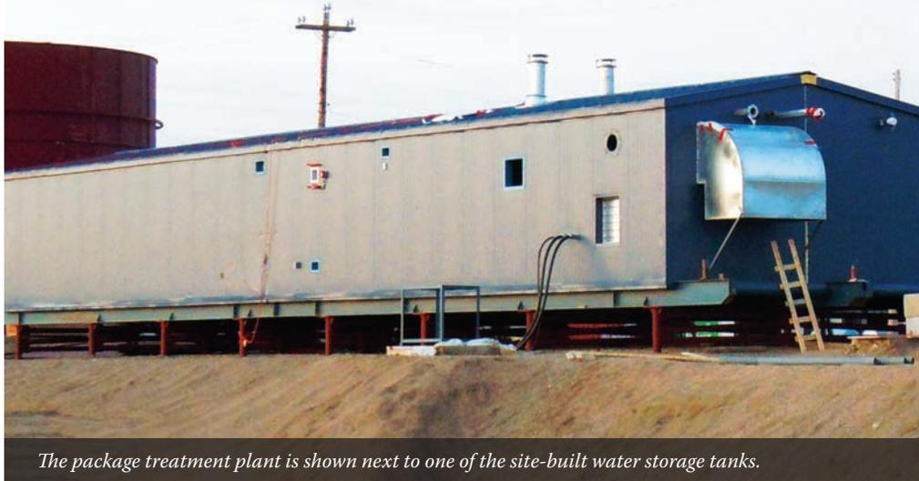
The package treatment plant is shown next to one of the site-built water storage tanks.
