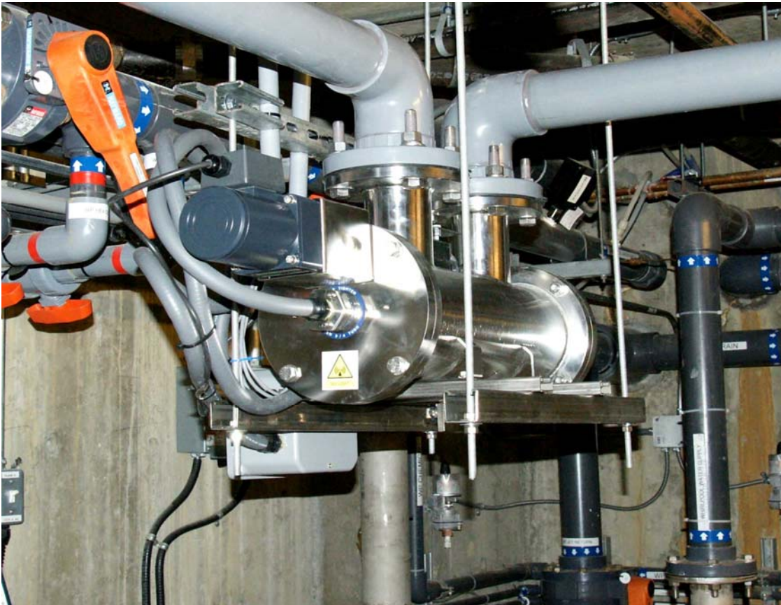
The Hanovia medium pressure UV unit can be installed in existing equipment rooms
