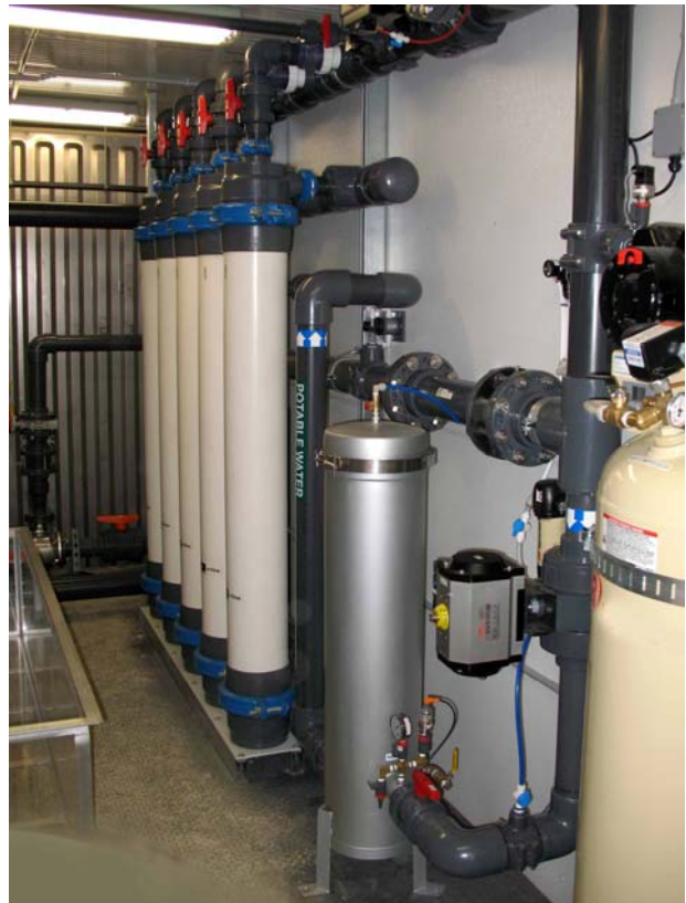
A 1 micron absolute filter follows the ultrafiltration membranes.
