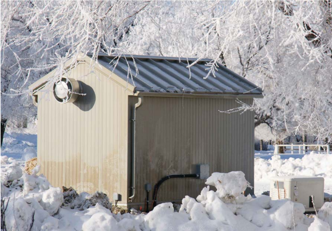
Completed Treatment Plant
