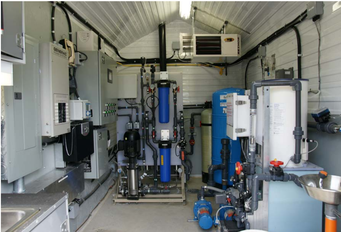
Interior of Water Treatment Plant
