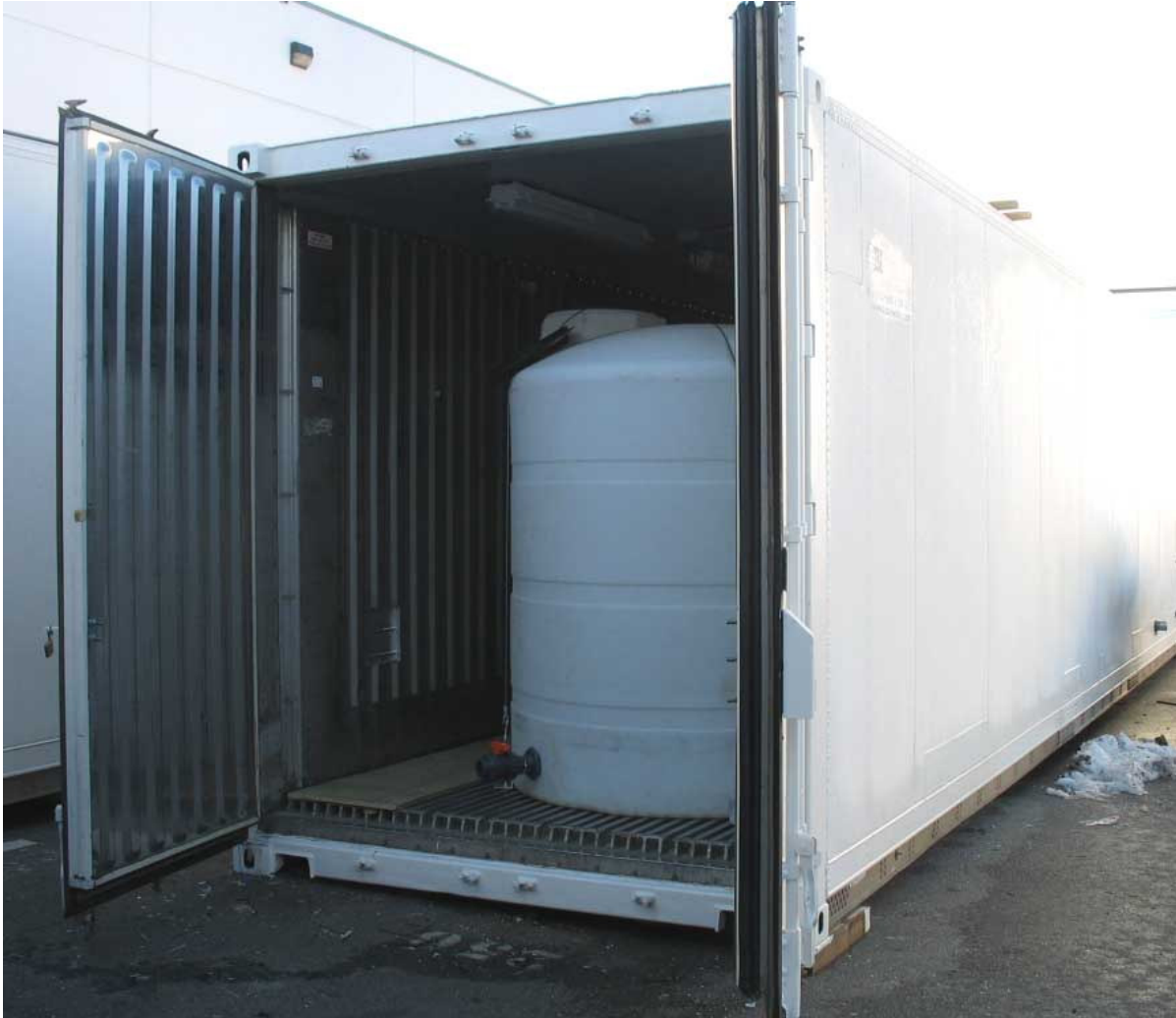
Water Treatment unit with treated water storage tanks in a 40 foot long insulated reefer
