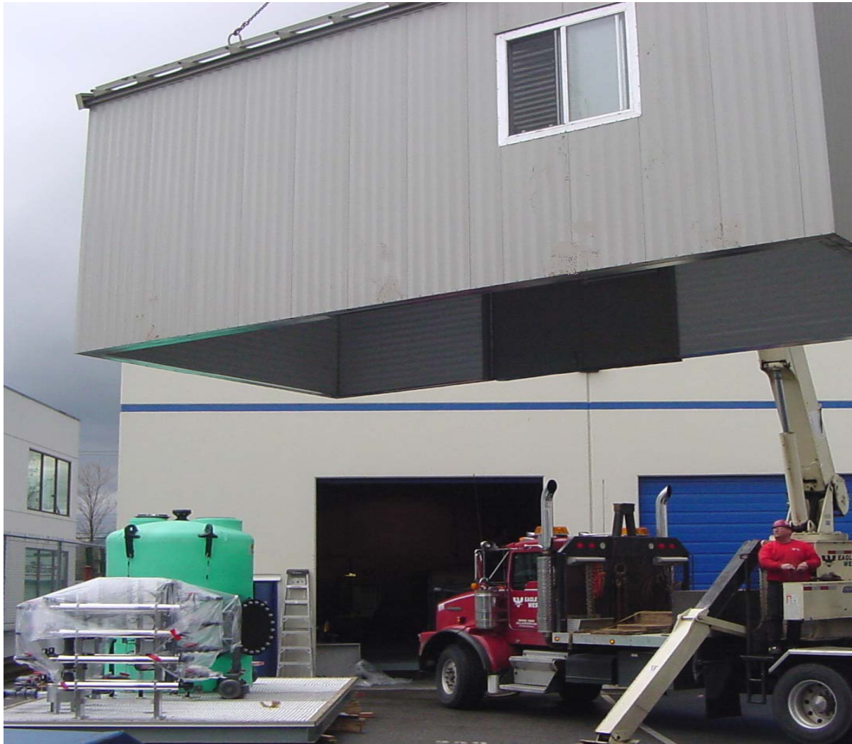
Lifting the water treatment plant building onto the skid.
