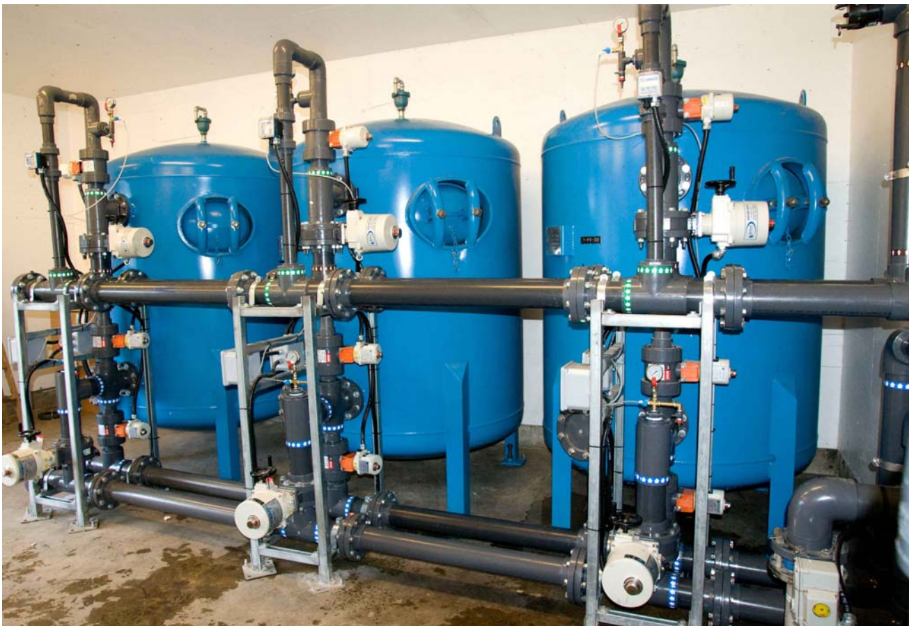
Figure 1 - FRP vessels with GreensandPlus media to remove Iron, Manganese, Hydrogen Sulfide, Arsenic and Radium.
